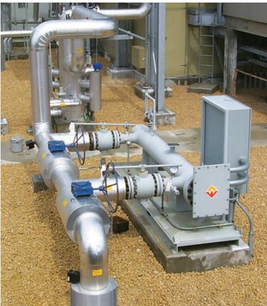
Fuel gas heater for a gas turbine
